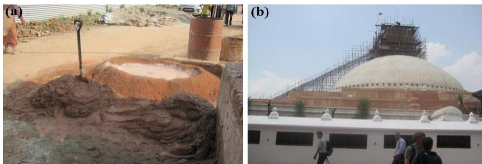
Figure 1. (a) Traditional Dyocha soil mortar replaced by the lime-mud mortar and (b) place for the yahsin has been taken by some new engineered element at Bouddha Stupa. (Source: From the Facebook post of Dr. Sudarshan Raj Tiwari)
